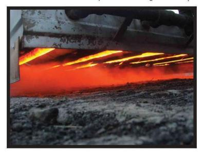
The same thermal technique is applied to cracks and existing saw cut joints.
